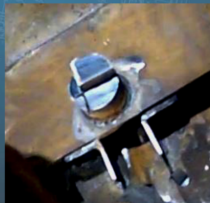
Step 2, Make horizontal cuts
